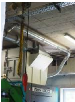
Photo 5: One thing that the shredder is short on – space. Vecoplan had to adapt the VIZ to the low ceiling.
