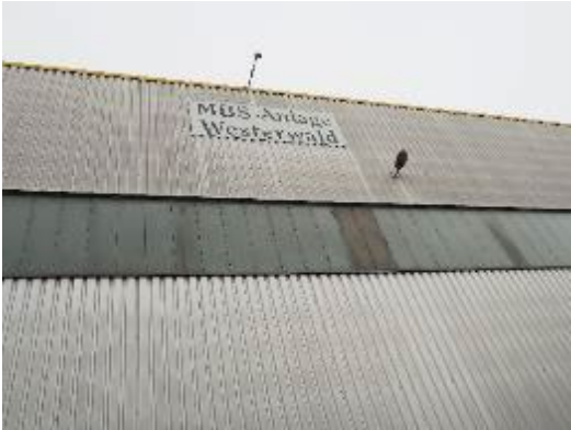
Photo 1: The MBS plant in Westerwald has been in operation since 2000. Vecoplan is the main supplier of processing technology for the company.
