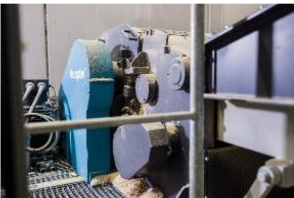
Photo 6: The drum chipper shreds the resulting waste wood to dryer-capable chip size.
